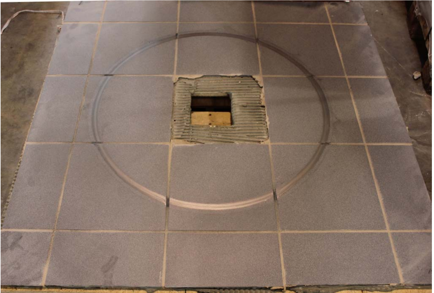
Image 1: Full assembly of the installed 12"x 12" Crossville Porcelain tile after testing (Figure 1)
